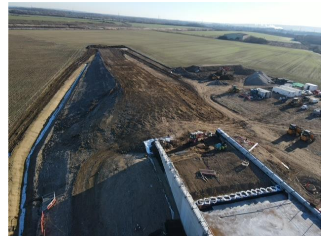
Embankment approach nearing completion
