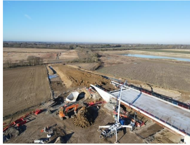
Waterproofing to bridge deck
