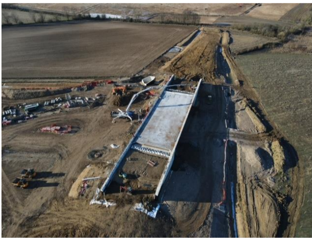
Completed bridge structure
